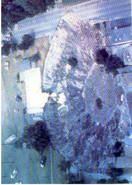
A collapse sinkhole that formed suddenly in Winter Park, Florida, in 1981
